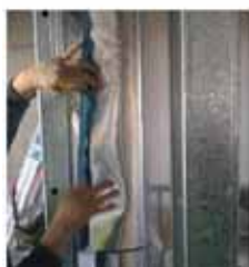
Wrap each segment with an overlap
